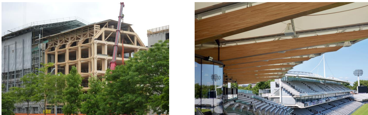
Slika 2. a) zgrada Tamedia u Zurich-u, LVL bukva [3]; b) Lord's Cricket Ground u Londonu, hrast [1]
